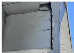
Repairs Dry Rot
