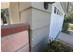
Repair Exterior Paint
