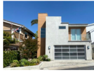
Front of Property
