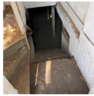
Stairs to Below House
